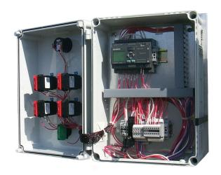
To ensure compliance with current NFPA requirements, Acme's Local Signal Panels provide a visual indication of an alarm condition.
